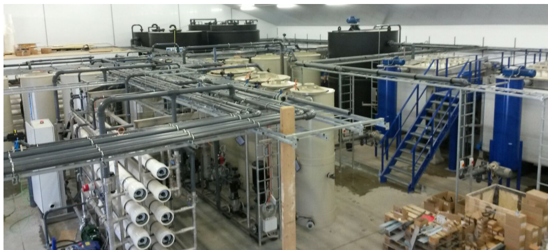
Figure 7. Membrane system. Photo: Regenisis.
