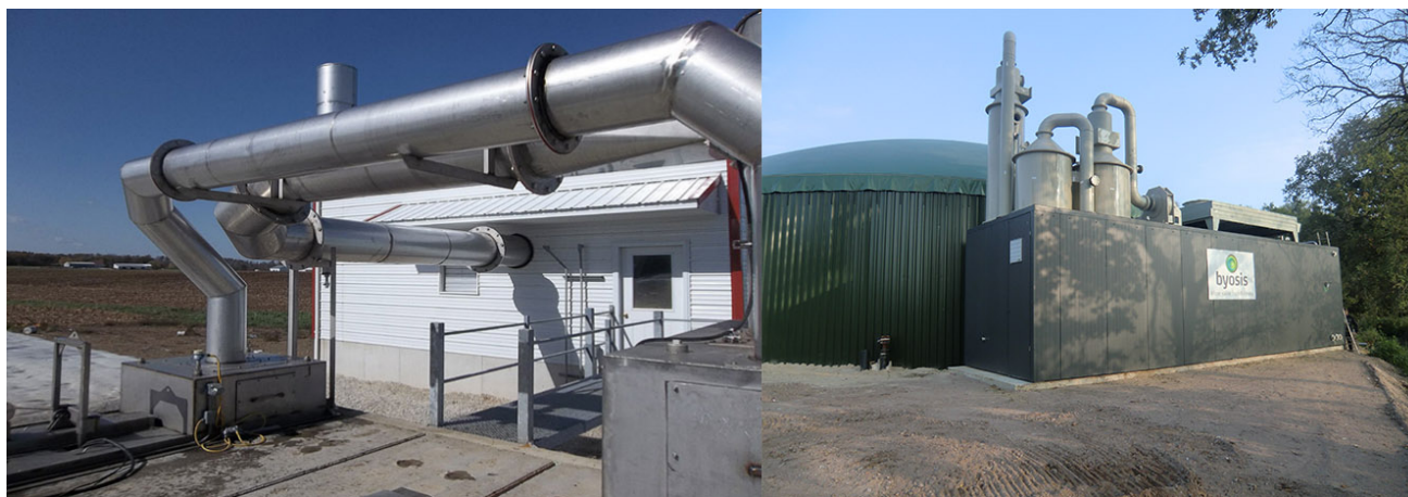
Figure 6. Non-chemical carbon dioxide and ammonia air stripper (left) and media tower ammonia air stripping (right). Photos: DVO Incorporated and Byosis.
